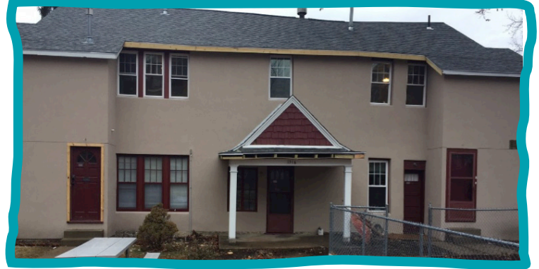
Carriage House After
